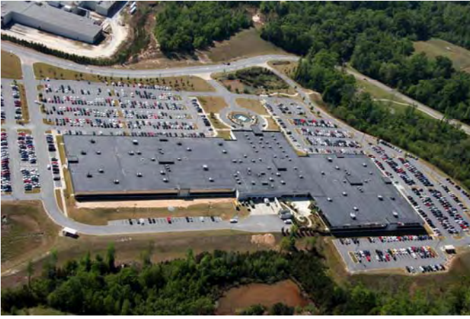
AFLAC Insurance Headquarters Columbus, GA 350,000 Square Feet Fully Adhered EPDM Single-Ply
