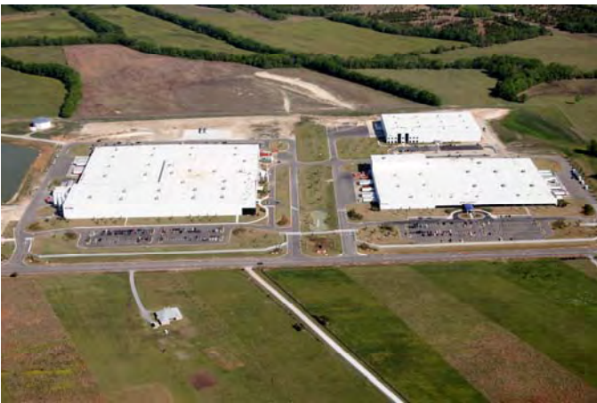
Mobis Alabama Burkeville, AL 700,000 Square Feet Mechanically Attached TPO Single-Ply
