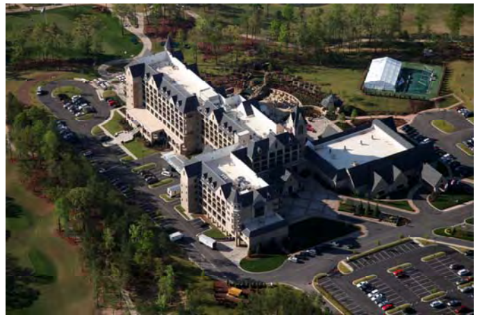
Ross Bridge Hotel Hoover, AL 85,000 Square Feet Plywood Decking/Underlayment 85,000 Square Feet GAF Slateline Shingles 69,000 Square Feet Fully Adhered TPO Single-Ply
