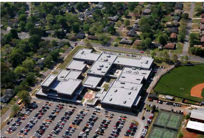
Huntsville High School Huntsville, AL 350,000 Square Feet GAF Modified Bitumen
