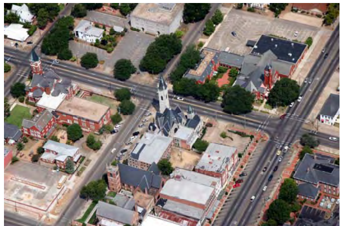
First Baptist Church Selma, AL 21,000 Square Feet Slate Shingles 26,000 Square Feet Terne Stainless Steel Roofing
