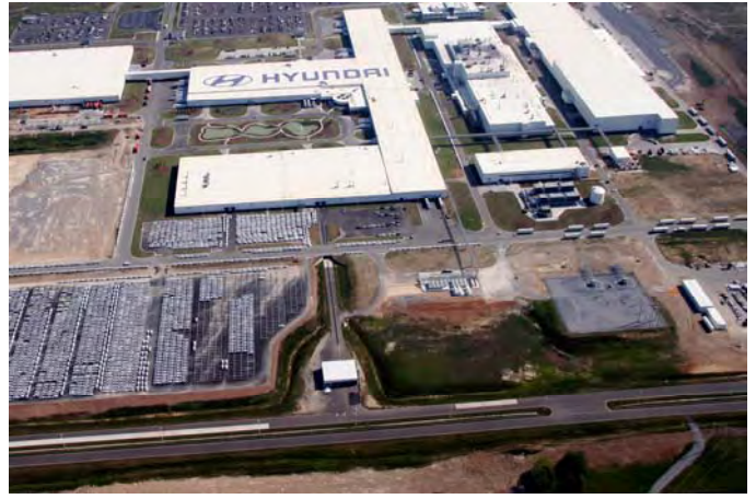
Hyundai Paint Shop Hope Hull, AL 320,000 Square Feet Mechanically Attached TPO Single-Ply
